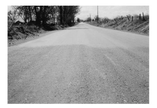
Photograph 1 shows the tightening and densifying effect of a rejuvenator treated pavement. (State of Idaho)
