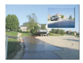
CRF® provides pavement rejuvenation as well as sealing the pavement surface, unlike standard asphalt emulsion that hardens and becomes brittle. CRF® was designed to be a corrective maintenance product that effectively repairs cracks as a "cold pour crack filler" in concentrated form and provides a pavement "restorative seal" when applied in diluted form.
