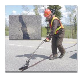
**CRF® Restorative Seal** is a petroleum oil and water cationic emulsion. Unlike standard asphalt emulsion, CRF® does not harden or "dry out" Designed as a one component emulsion that effectively repairs cracks in concentrated form, CRF® provides a excellent pavement restorative seal when applied in diluted form.
